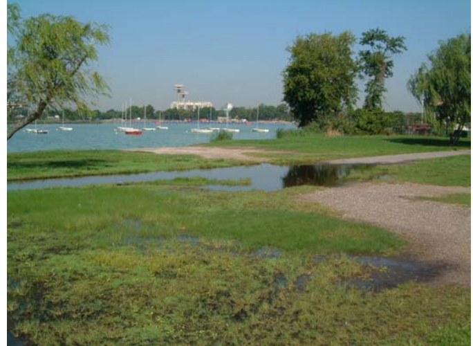
In a number of cases, failed pumps, or modified water tables emerge next to or over infrastructure, created more or less permanent wetland features – havens for mosquitoes in summer and ice hazards in winter.
